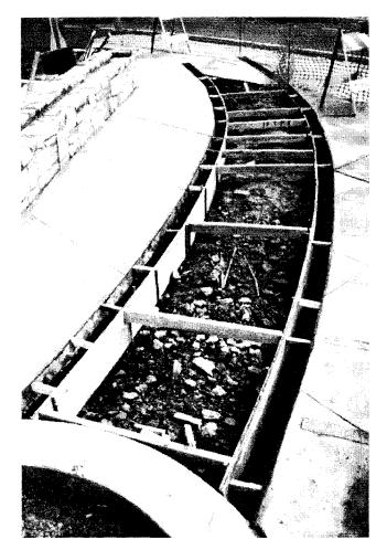
Fig. 8. Formwork during construction of the concrete rails.
